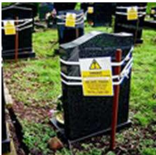
Temporary support systems will result in the delay of the primary inspection as time and resource has to be spent on the regular re-inspection of the 'make-safes' to ensure they remain safe should they remain for a long period. It is recommended that temporary supports remain for 3 months which gives the owner sufficient time to make arrangements for repair
